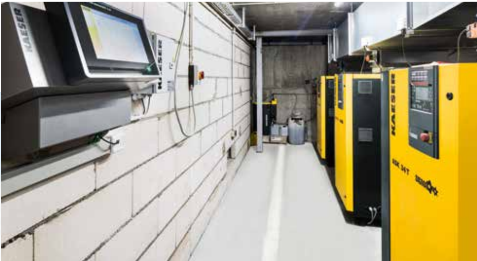
The advanced compressor system is monitored by a SIGMA AIR MANAGER 4.0 master controller
