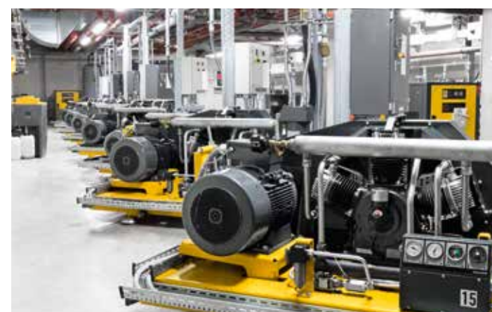
Top: 10-bar compressor station with rotary screw compressors Bottom: 45-bar compressor station with booster compressors
