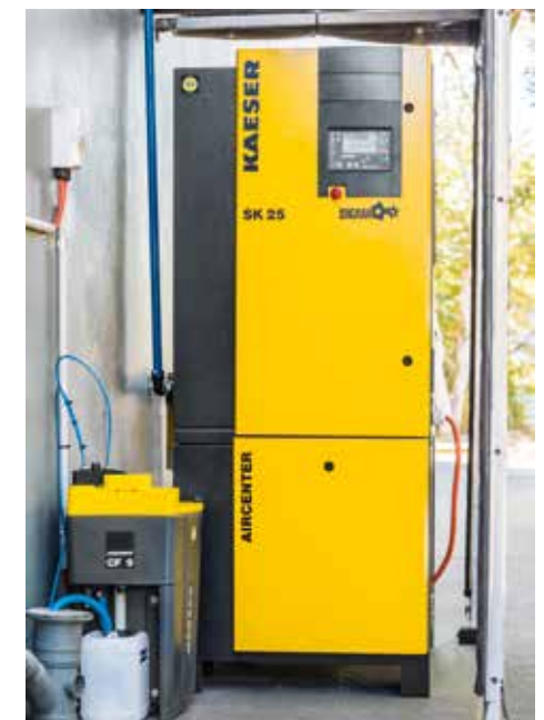
Bright Print replaced an outdated compressor with a new KAESER AIRCENTER SK 25
